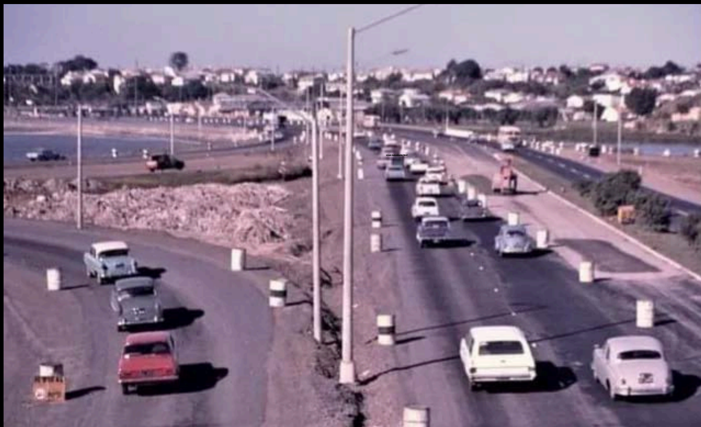
Onewa Road, Northern Motorway 1968
