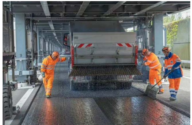
Work takes place under the bridge
