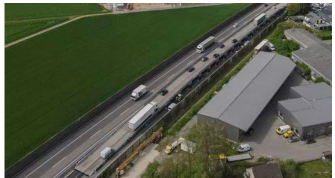
An Aerial view of the new bridge
