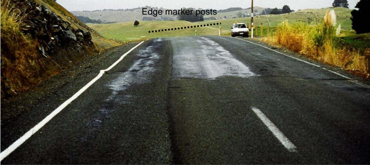
Figure 5 Edgeline, centreline and edge marker posts
