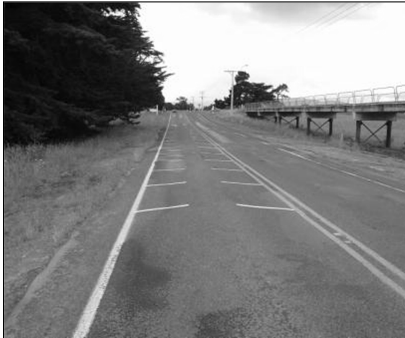
Photo 2: Trial Site 1: State Highway 53
