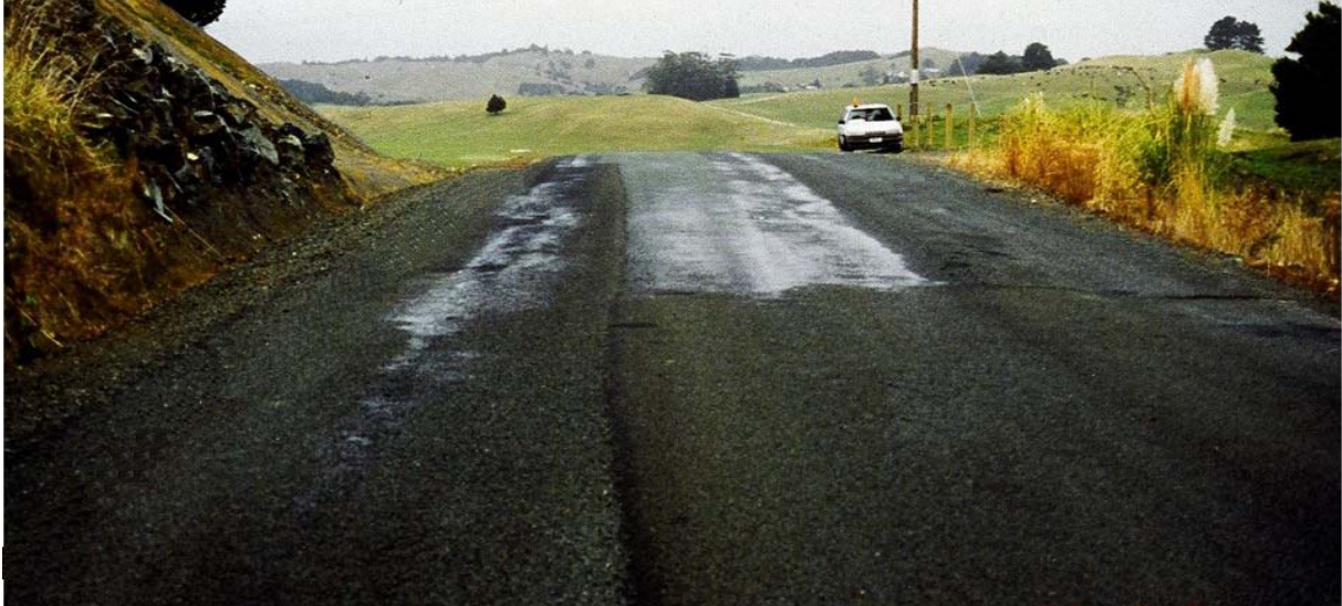
Figure 2 A section of low volume rural road
