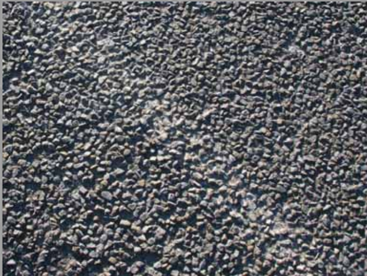
Road markings before (38RI)
