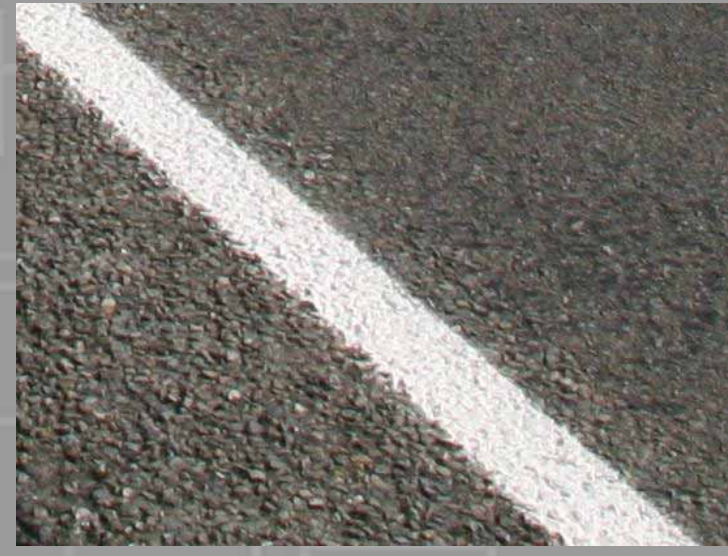
Road markings after (142RI)
