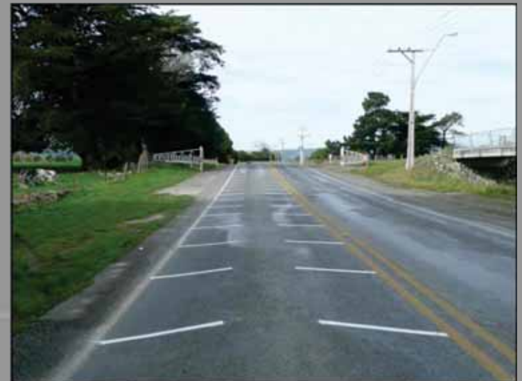
Transverse road markings – Before and after Andrew Martindale
