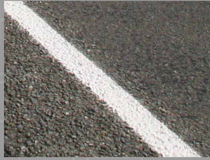
Road markings after (142RI)
