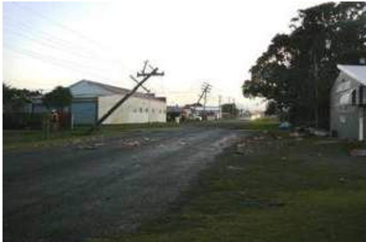
Wind damage, Opunake Taranaki 22 July 2009
