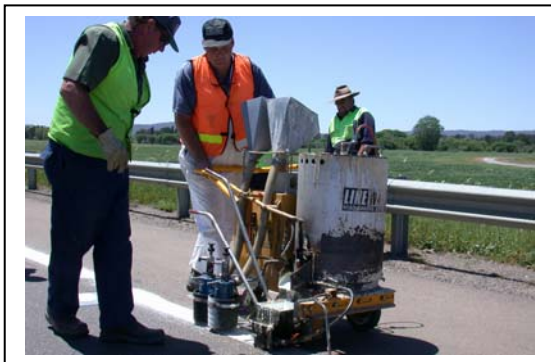
Above: Lineways application equipment, used to apply the thermoplastic markings.
