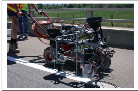
Above: TCP application equipment, used to apply the PMMA two-component cold applied plastic markings.
