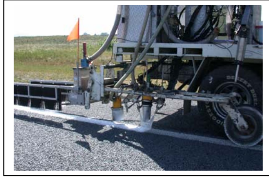
Above: Potters application equipment, used to apply the waterborne 3427 Fastrack markings.
