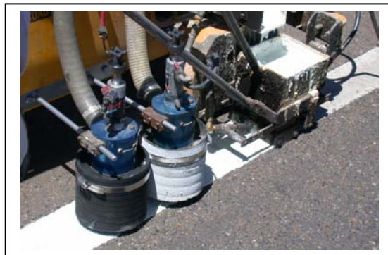
Above: Lineways application equipment, used to apply the thermoplastic markings.
