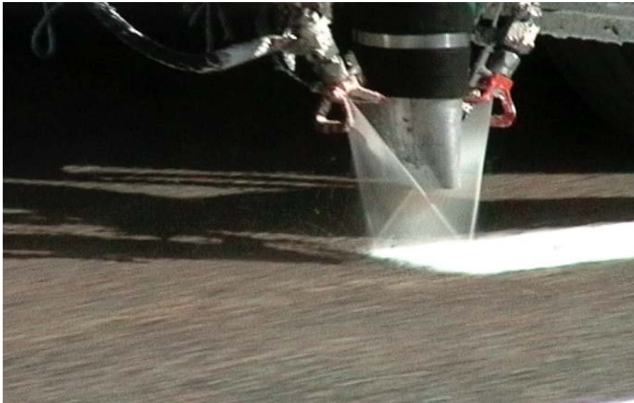
Encapsulation method for applying angular particles into PMMA.
