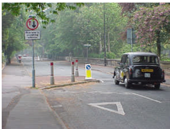
A chicane & speed hump treatment in the United Kingdom.
